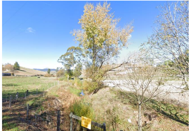
View south from Edward Street
